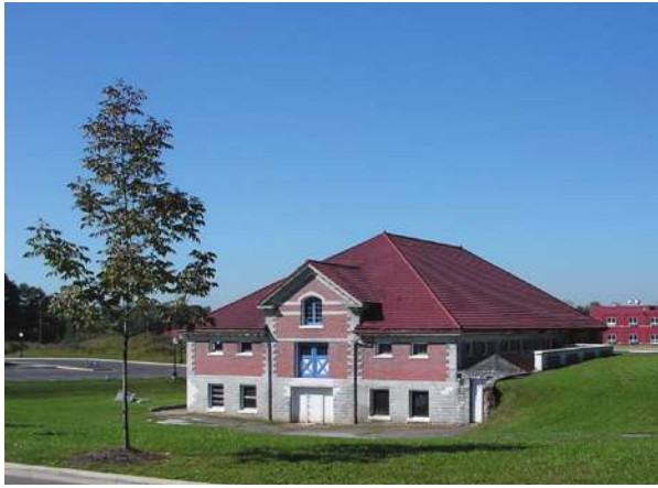
The Heating House
