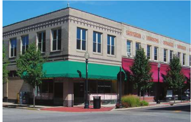
Tuscarawas Avenue Commercial
