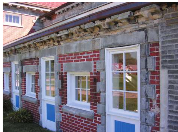
The Piggery Restoration
