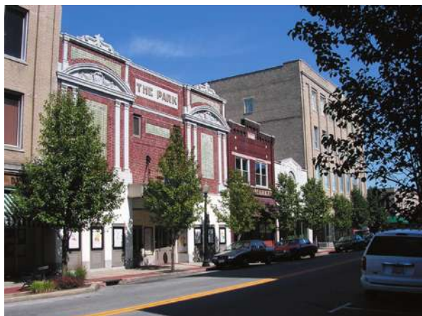
Tuscarawas Avenue Commercial
